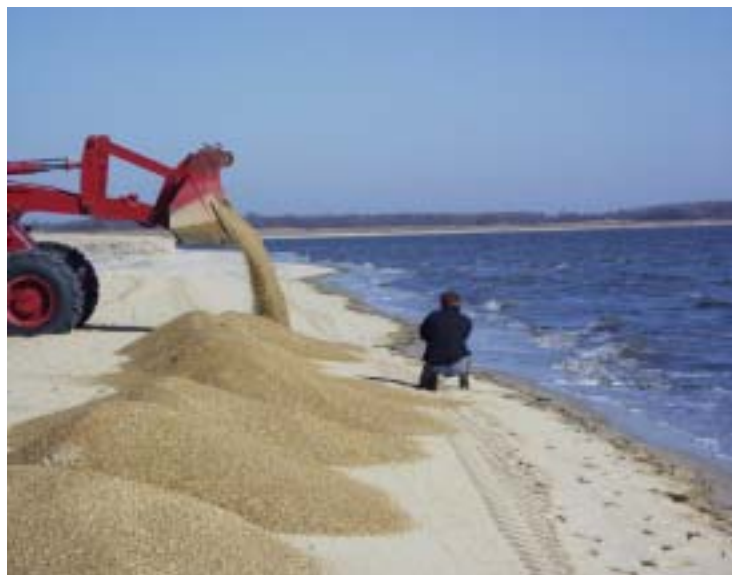
PEA GRAVEL BEING PLACED ON NORTH BOWERS BEACH, APRIL 2002
