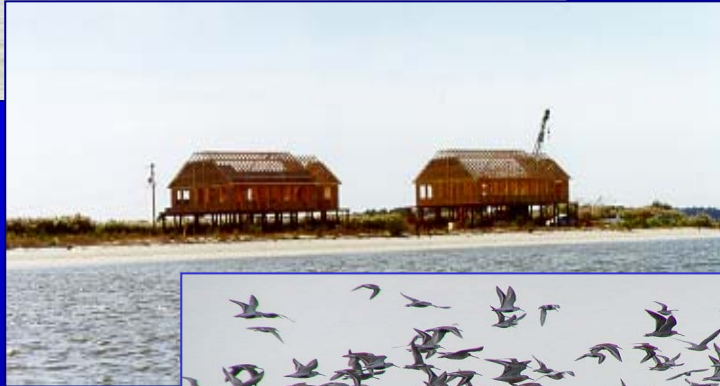
New Construction St. Jones River/Bowers
